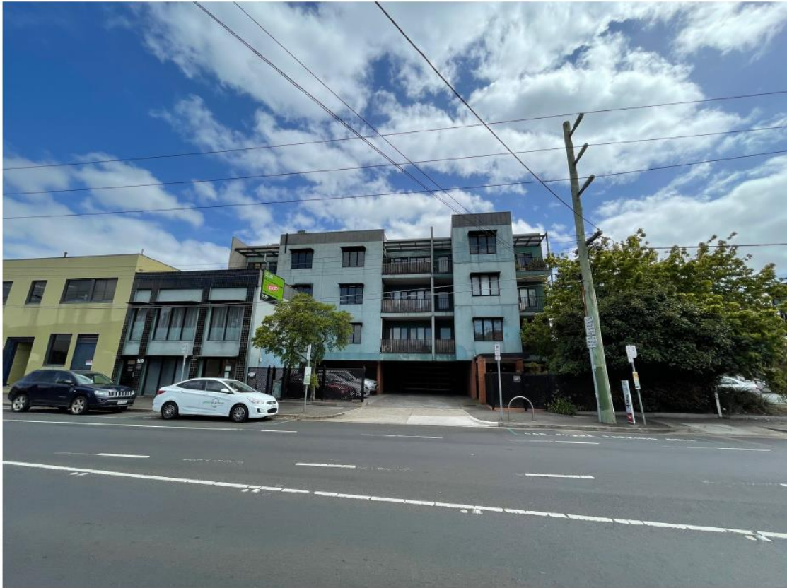
Extract from Dr Bunting's photographs showing the south row of apartments behind the two storey offices that have an outlook to Glenlyon Road.
